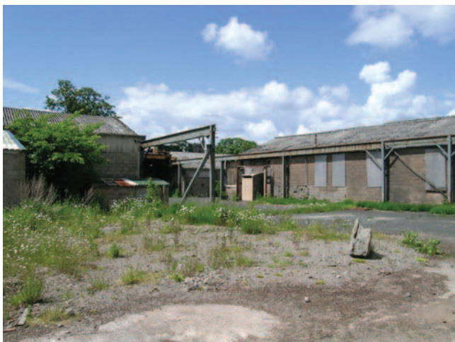
Cumbria Stoneworks site. Courtesy of Lyvennet Community Trust
